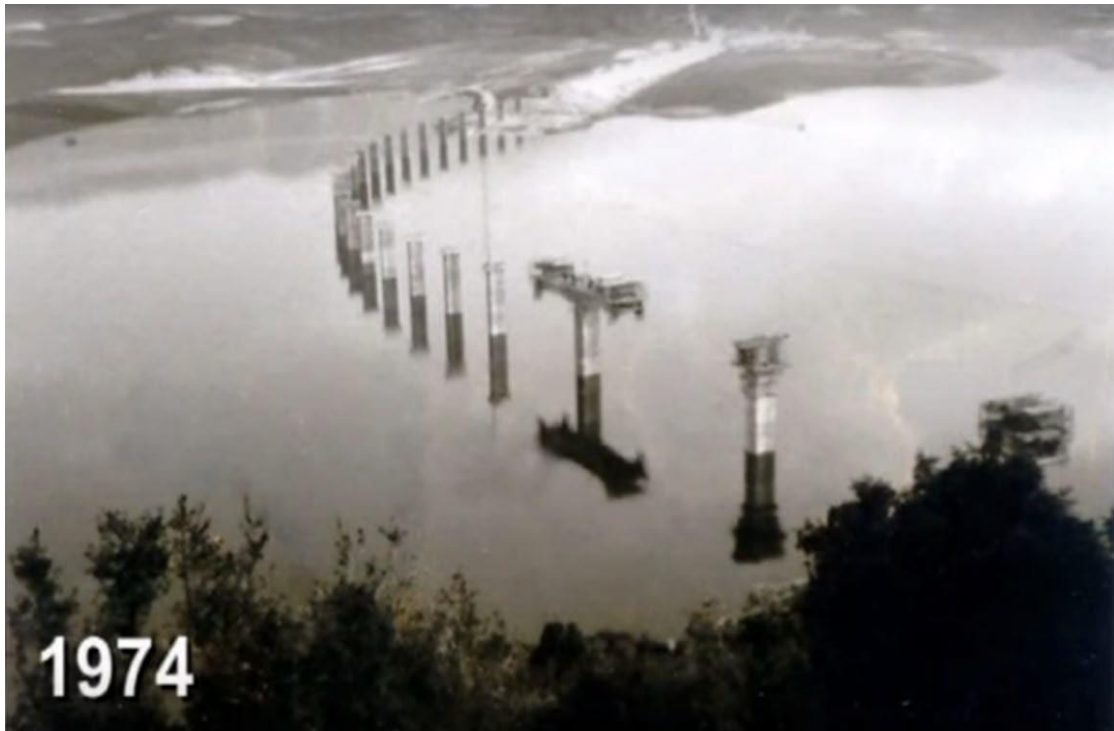
Figure S7. Impoundment of Neraida village and construction of the approximately 1500 meters Polyfyto Bridge.
